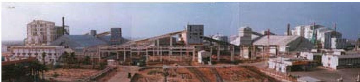
IFFCO Kandla Unit – NPK/DAP Complex. Production Capacity NPK/DAP 2.42mtpa
