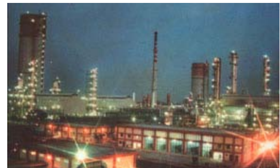
IFFCO Anola Unit – Ammonia-Urea Complex. Production Capacity Ammonia 1.003mtpa; Urea 1.730mtpa
